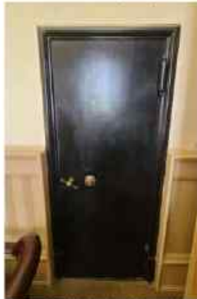
Image 94 – Vault door at Level 4, Room 104
