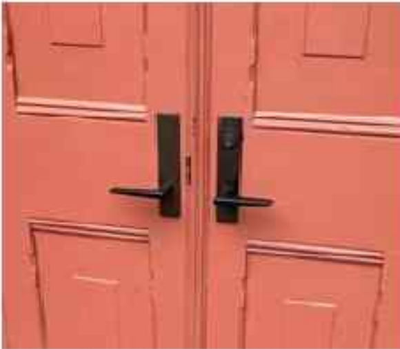
Image 58 - Modern hardware levels at ADA accessible entry
