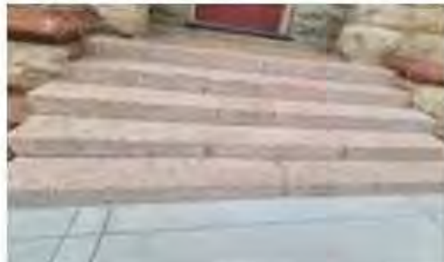
Image 67 - Granite steps leading up to the north porch
