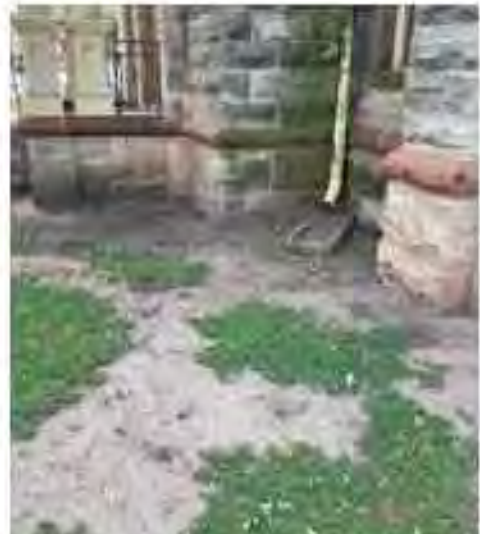
Image 15 - Typical downspout termination at splash block.
