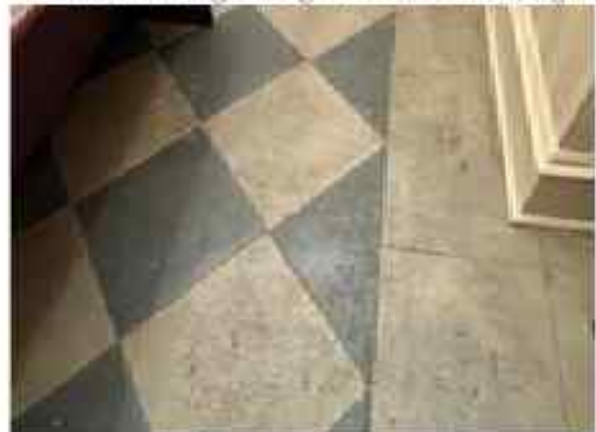
Image 70 - Historic scored concrete at 1st Floor
