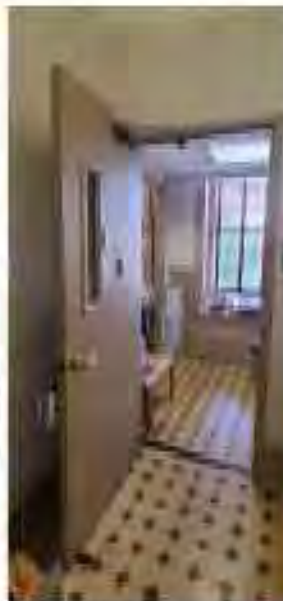
Image 88 - Metal door in Room 202
