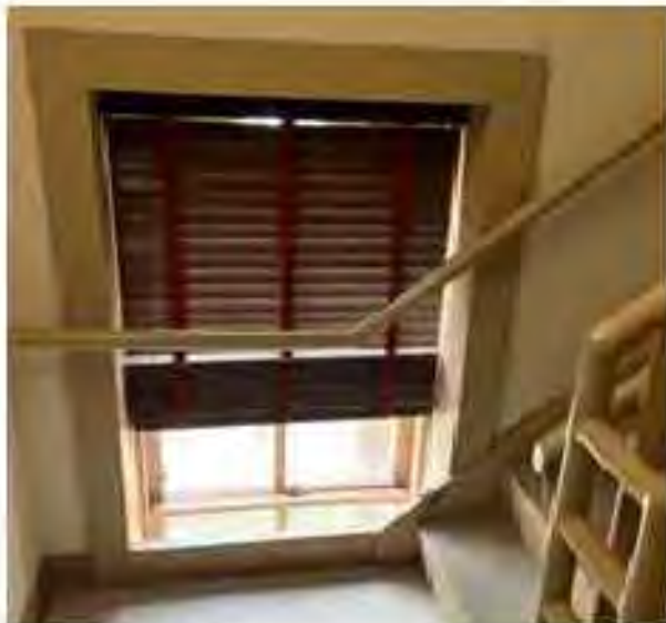
Image 99 - Window in staircase
