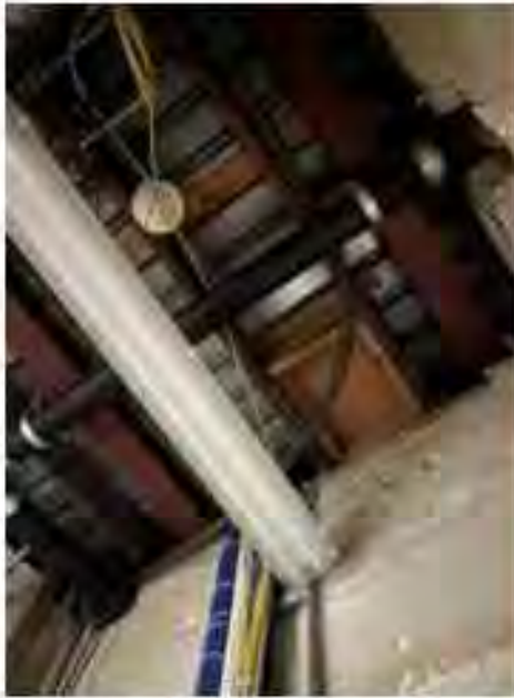
Image 124 - Underside of existing structural bay adjacent to elevator tower
