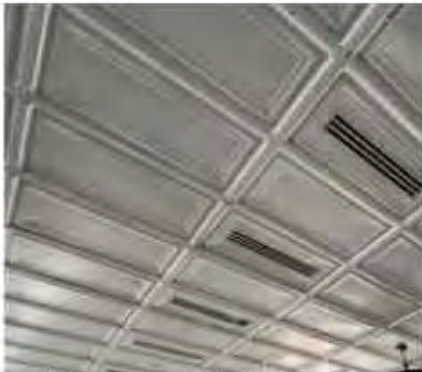
Image 77 - Courtroom pressed metal ceiling
