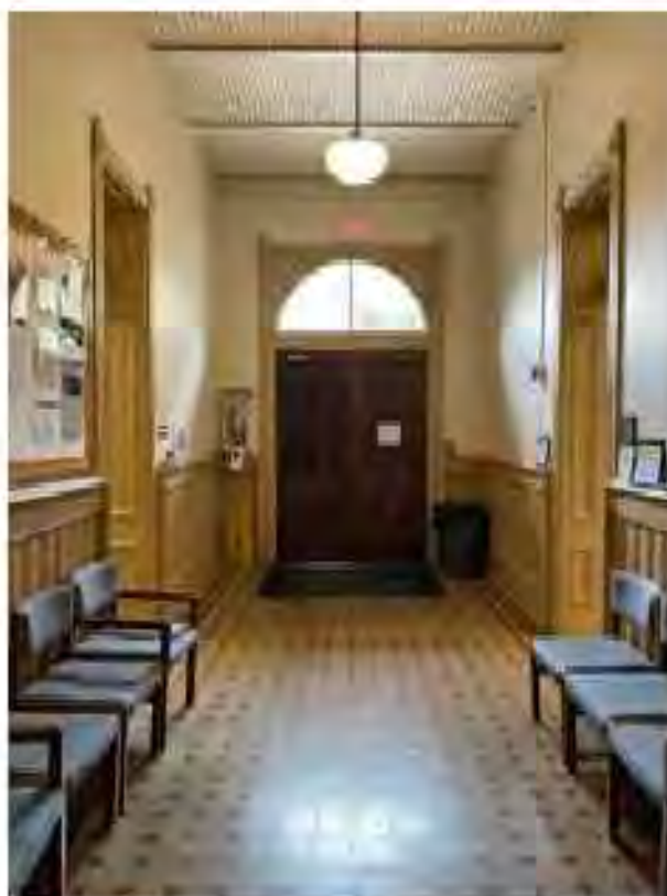
Image 3 – Typical Interior Corridor
