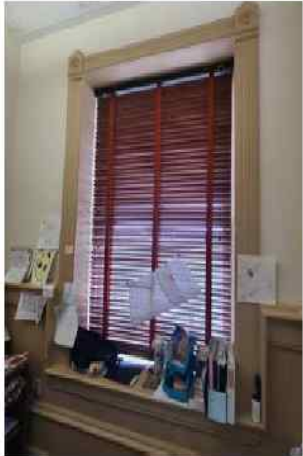
Image 57 - Typical painted window
