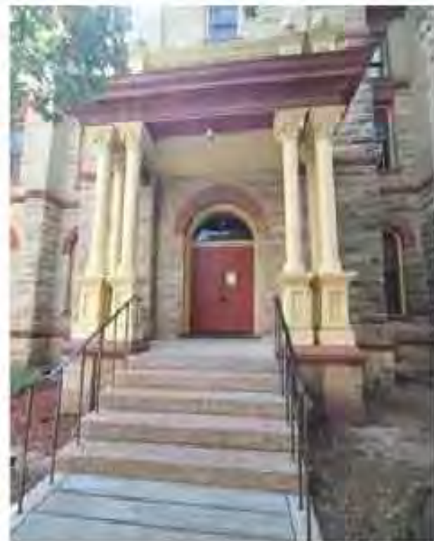
Image 36 - East entry porch
