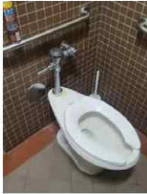
Image 141 - Existing water closet and flush valve
