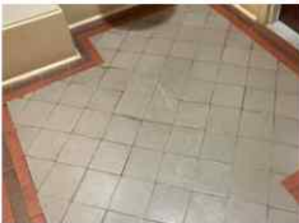
Image 75 - Typical tile in Elevator Lobby & in sections of the 2nd Floor Corridor
