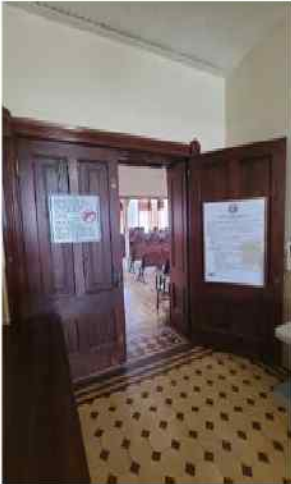
Image 91 – District Courtroom Entry doors
