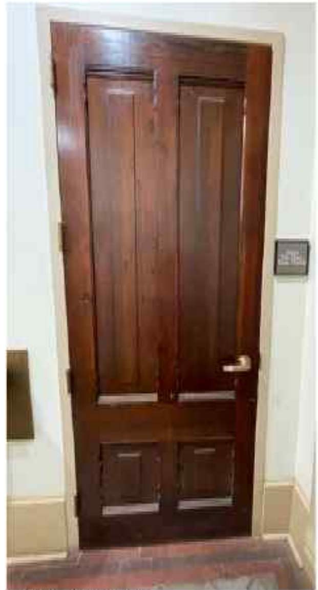
Image 92 – Typical fire stair door
