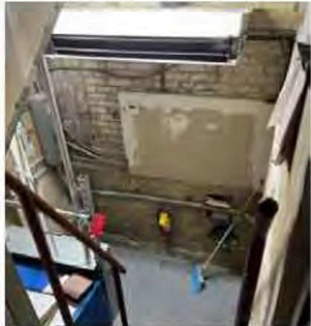
Image 122 – Partial Basement adjacent to elevator shaft area room.
