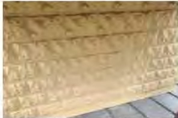
Image 49 - Metal cladding at mid-height to look like stone
