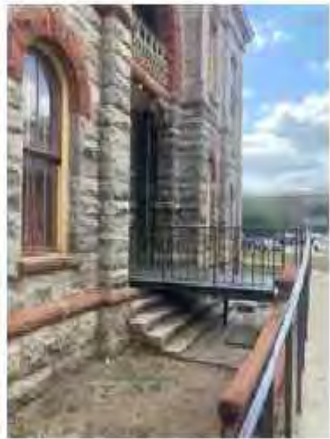
Image 33 – Accessible ramp at north porch.
