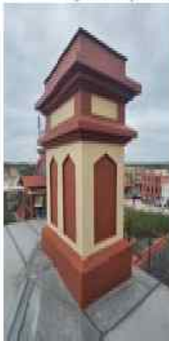
Image 50 - Typical chimney conditions
