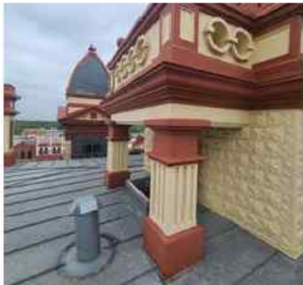
Image 46 - Standing seam metal main roof and base of clock tower on main roof.
