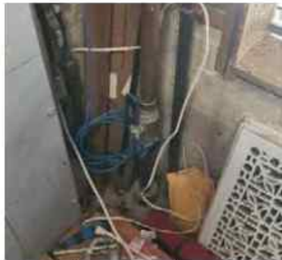
Image 142 - Domestic water entry to partial basement
