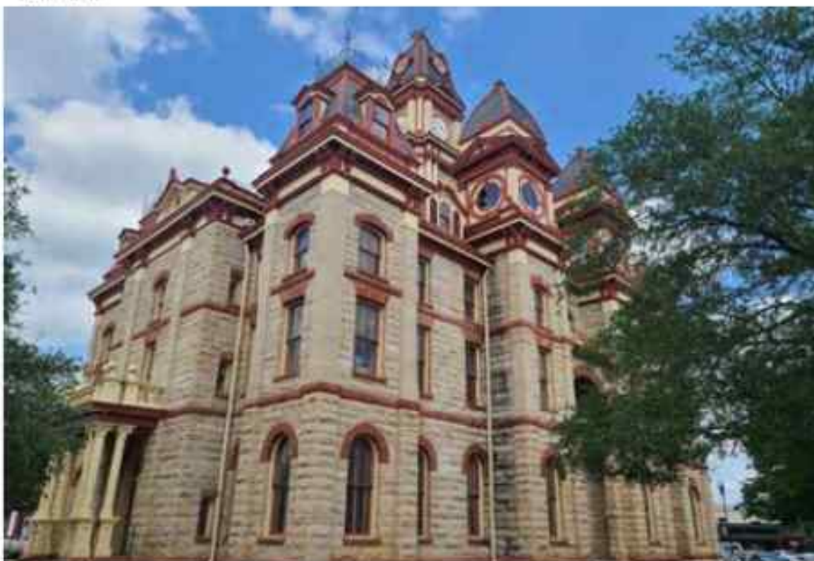
Image 3 - Southeast corner of courthouse
