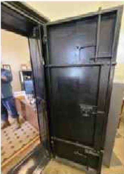
Image 93 – Interior of vault door at Level 3, Room 101 (Tax Office)
