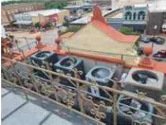
Image 47 - HVAC units & oil canning of metal on lower roof
