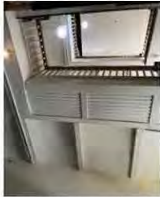
Image 125 - Underside of existing structure at second floor stair opening
