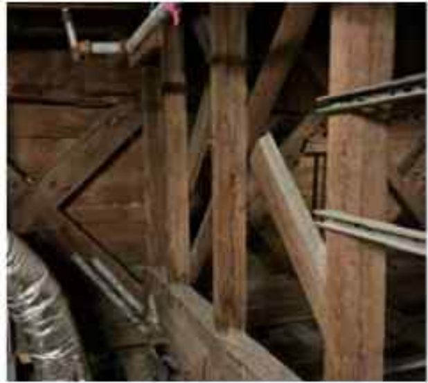
Image 133 - Wood framing at roof framing and existing wood roof deck.
